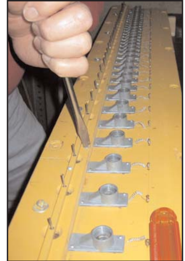
Figure 58. The valve cover is on the left.
