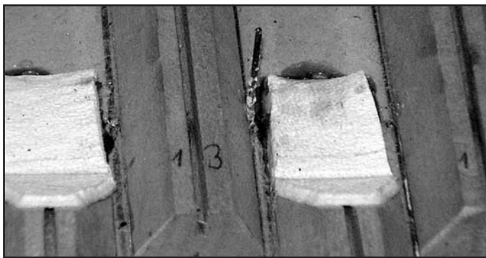
Figure 9. Pallet guide pins showing corrosion and general poor condition.
